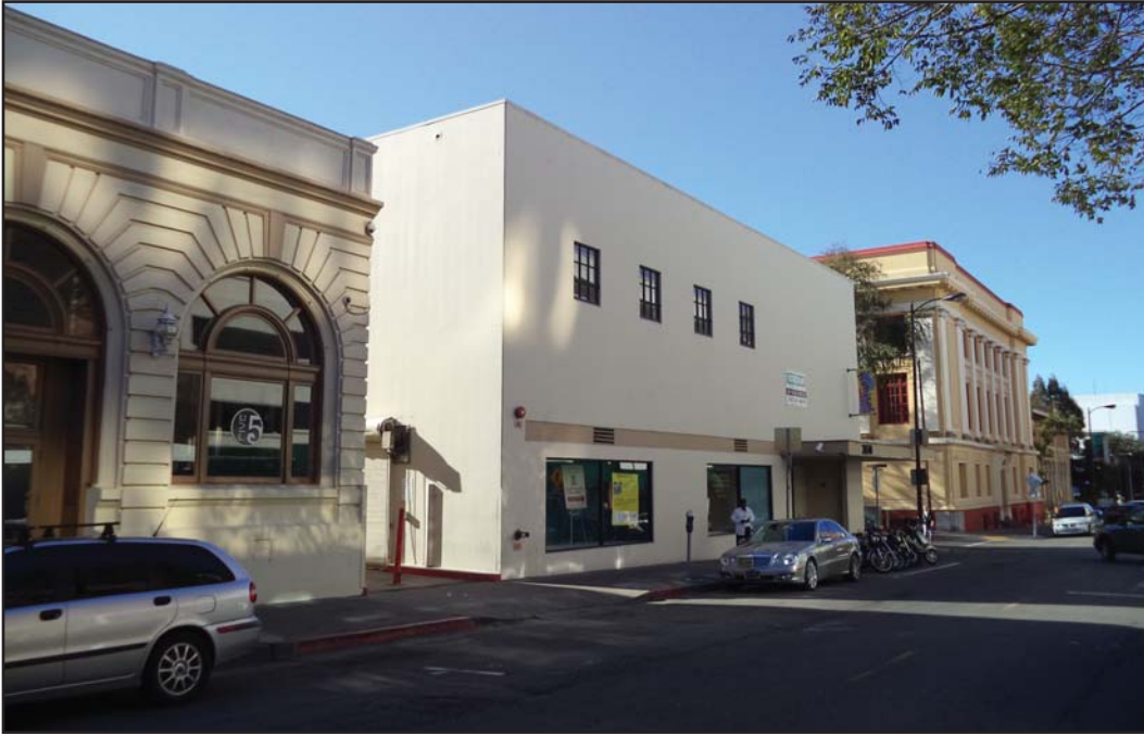
Photo 1 - View of the Allston Street frontage of the existing “Postal Annex” building, also known as the 1958 Hink’s Building, at the corner of Harold Way and Allston Way, looking southwest from across Allston Way. The adjacent one-story 1912 Restaurant Addition portion of the Shattuck Hotel is visible to the left of the frame, and the Dharma College building across Harold Way from the site is visible in the right of the frame.
