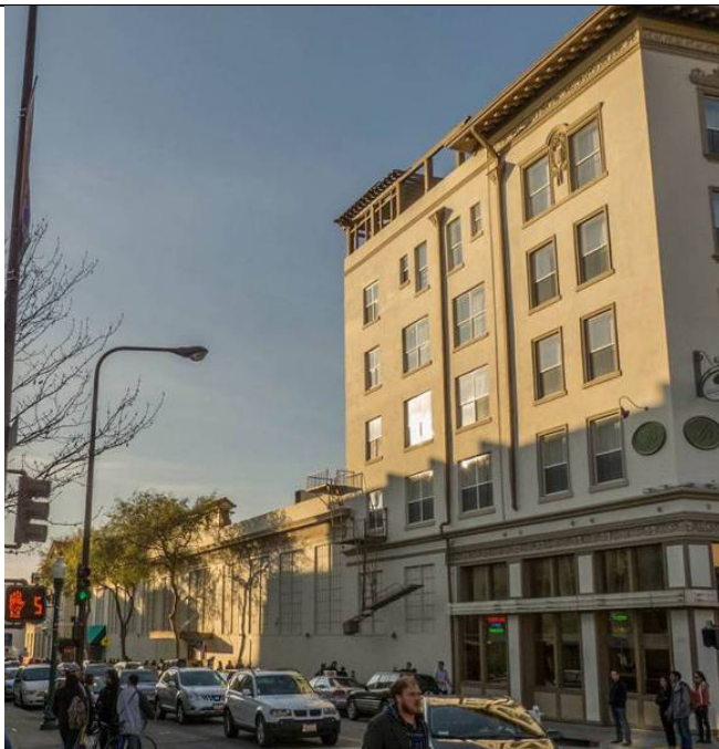
South (Kittredge Street) elevation, view looking roughly northwest from Shattuck (Architectural Resources Group, December 2013)
