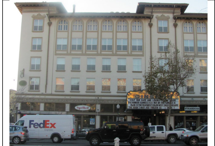
Current cinema entrance at south end of east elevation, former Hink's Department Store entrance (Architectural Resources Group, December 2013)
