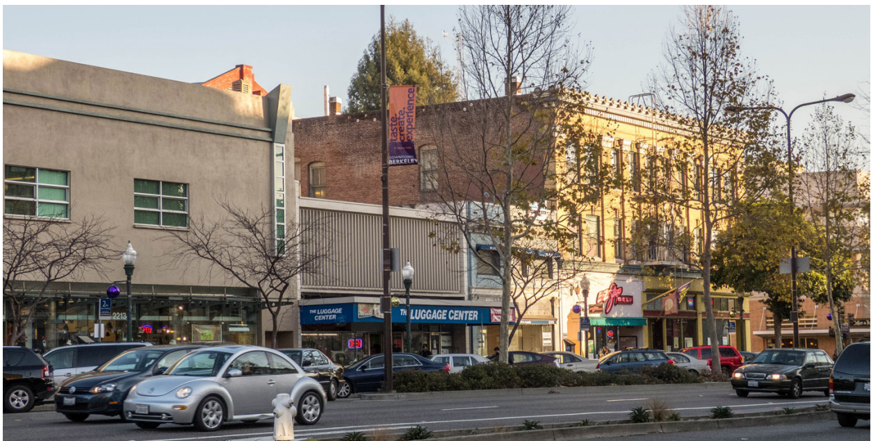
Looking southeast from Allston Way and Shattuck Hotel block at buildings along east side of Shattuck Avenue (2200 block) (Architectural Resources Group, December 2013)
