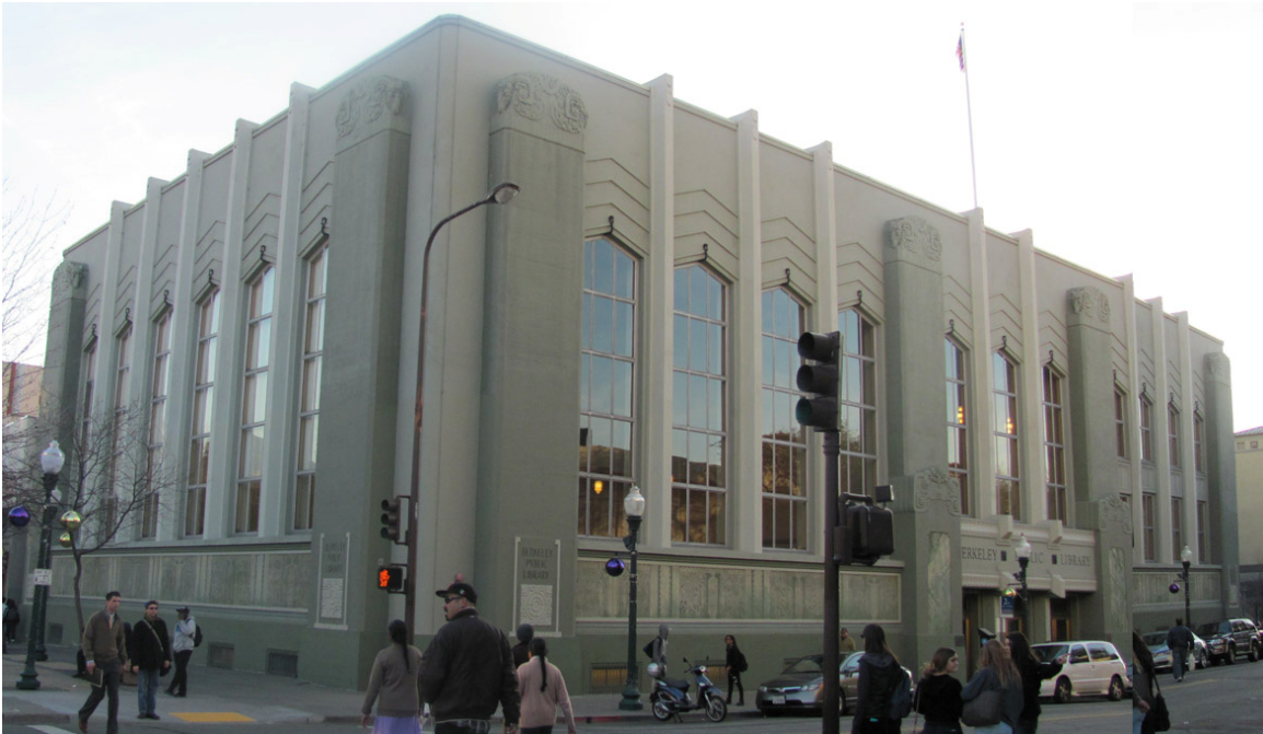
Berkeley Library, 2090 Kittredge St. (photo composite), looking southwest from Shattuck (Architectural Resources Group, December 2013)
