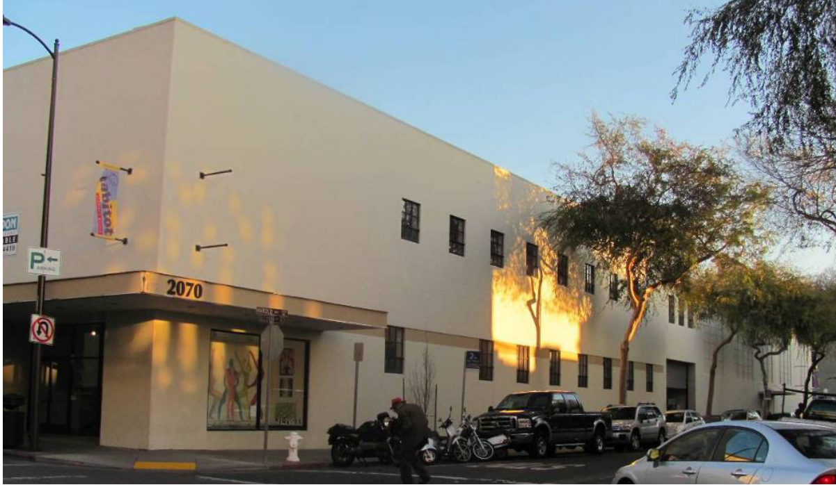
West (Harold Way) elevation, view looking southeast from Allston Way, 1959 addition in foreground (Architectural Resources Group, December 2013)
