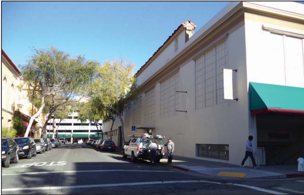
Photo 3 - View of the Harold Way frontage of the Shattuck Cinemas building, also known as the 1926 Hink's addition to the Shattuck Hotel, looking north from across Kittredge Street.
