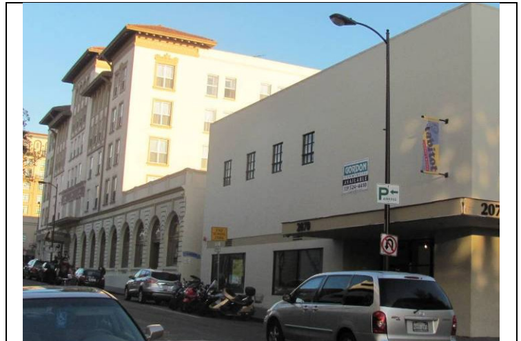
North elevation, view looking east across Allston Way, 1959 addition in foreground (Architectural Resources Group, December 2013)
