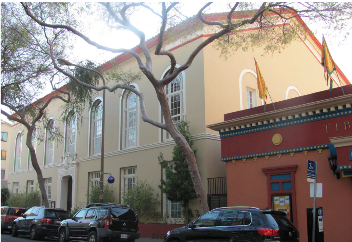
Dharma Institute, 2222 Harold Way, looking southwest across Harold Way (Architectural Resources Group, December 2013)
