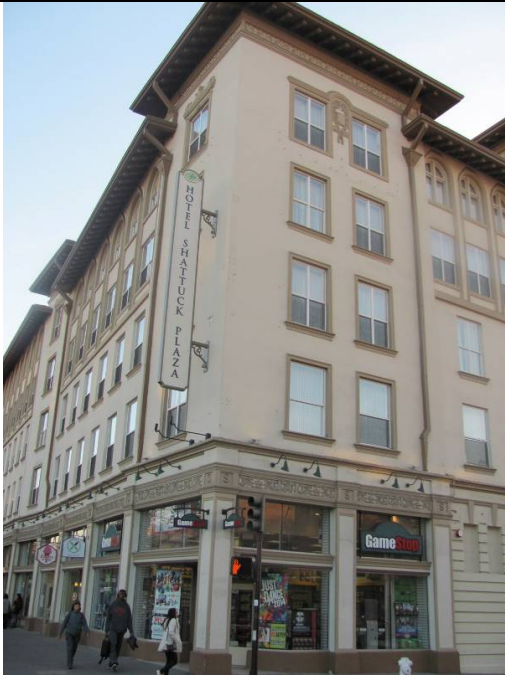
Detail of northeast corner, Shattuck Hotel (Architectural Resources Group, December 2013)
