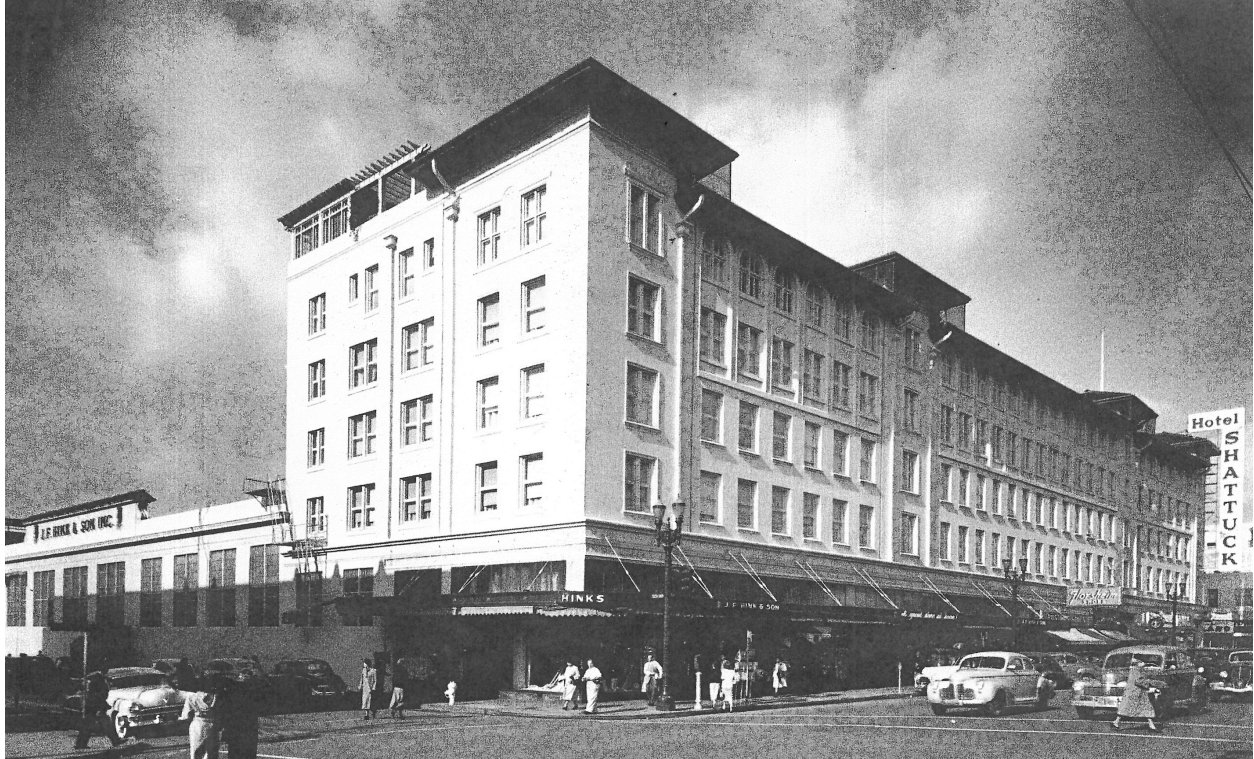
Shattuck Hotel, c. 1930, showing rear 1926 addition to hotel (Source: Berkeley Historical Society).
