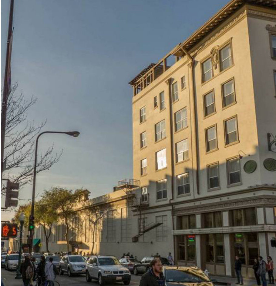
South (Kittredge Street) elevation, view looking roughly northwest from Shattuck (Architectural Resources Group, December 2013)
