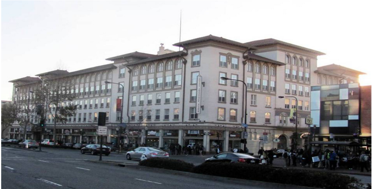
East (Shattuck Avenue) elevation and north (Allston Way) elevations, view looking southwest across Shattuck (Architectural Resources Group, December 2013)
