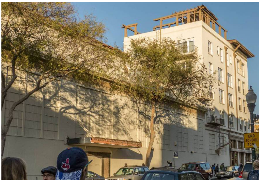
South elevation, view looking roughly northeast from across Kittredge (Architectural Resources Group, December 2013)
