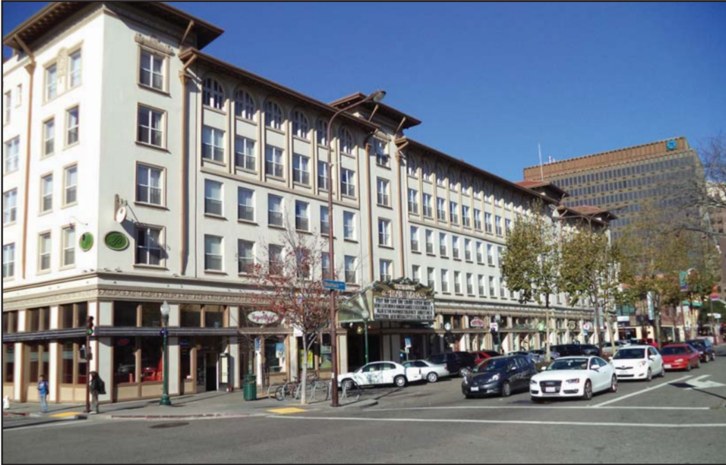
Photo 7 - View of the Shattuck Hotel building, immediately adjacent to the project site, looking northwest from across Shattuck Avenue.
