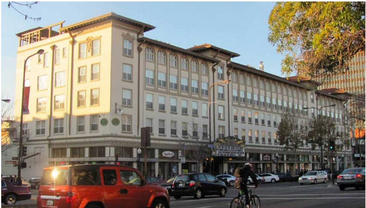
East (Shattuck Avenue) and partial south (Kittredge Street) elevations, view looking northwest across Shattuck (Architectural Resources Group, December 2013)
