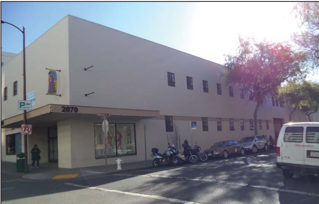
Photo 2 - View of the corner and the Allston Way and Harold Way frontages of the 1958 Hink’s Building looking southeast from across Allston Way.
