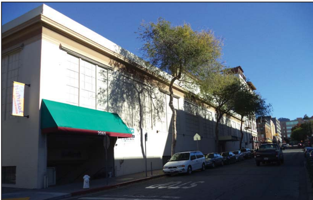
Photo 4 - View of the Kittredge Street-fronting portion of the 1926 Hink's Addition/Shattuck Cinemas building looking northeast from across Kittredge Street.
