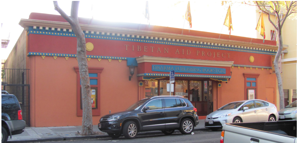
Tibetan Aid Project/Dharma Publishing Bookstore, 2210 Harold Way, looking roughly west across Harold Way (Architectural Resources Group, December 2013)
