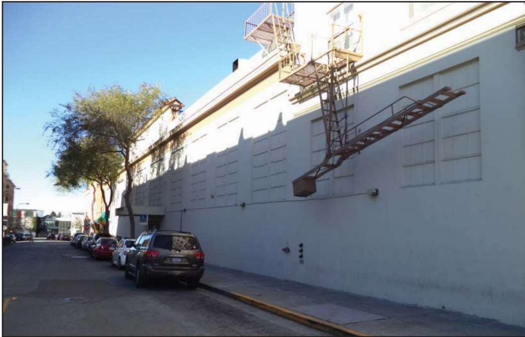
Photo 5 - View of the Kittredge Street-fronting portion of the 1926 Hink's Addition/Shattuck Cinemas building looking west from Kittredge Street.
