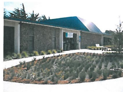
Figure 5-2: Bioretention area, Daly City (example of a flow-based treatment measure)
